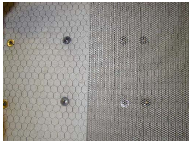
(6) INSTALL 4720-09 PERFORATED METAL And 2006-00 SPEED CLIPS (Fastener)
