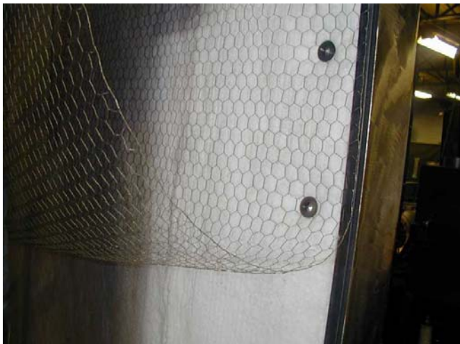
(5) INSTALL 2400-00 SS HEX MESH WIRE
