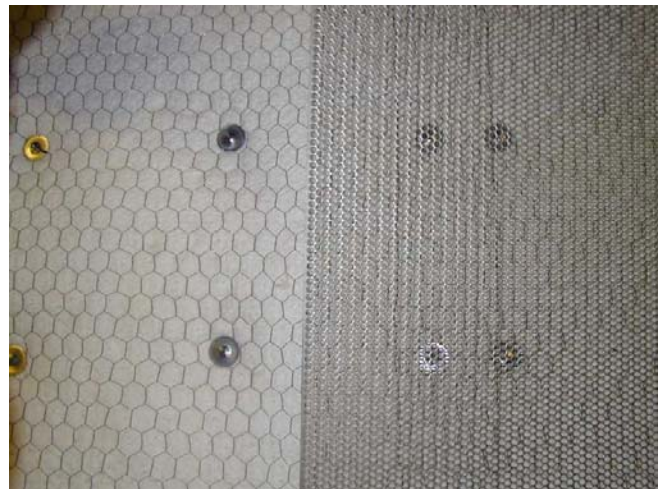
(6) INSTALL 4720-09 PERFORATED METAL And 2006-00 SPEED CLIPS (Fastener)
